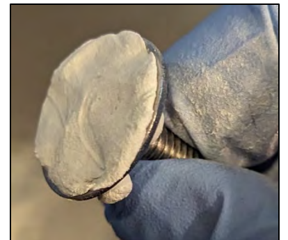
Figure 10: Completely cover bottom surface of stud with mixed epoxy
