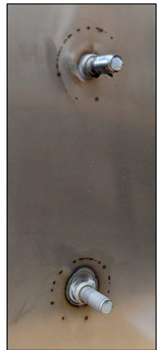
Figure 3: Included studs welded to tank
