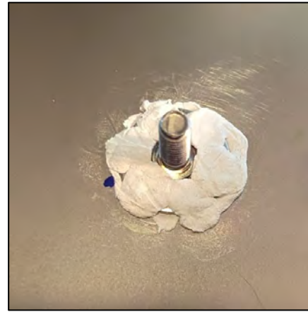
Figure 11: Evenly distribute the epoxy across the top of the stud base
